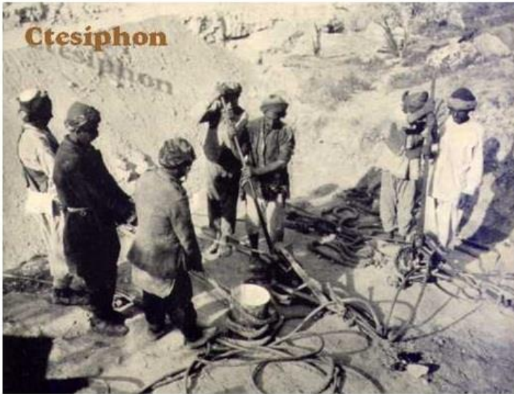
Trewhella Winch Operators controlling bridge erection
